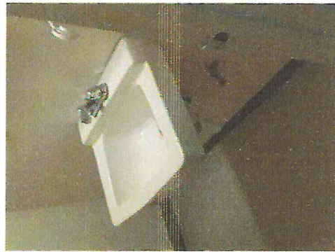
Building: Suite A 2511, Room: 27 Toilet Room, Element Id: LAV1-01
