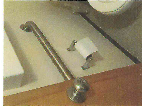
Building: Suite A 2511, Room: 27 Toilet Room, Element Id: GBSW1-01
