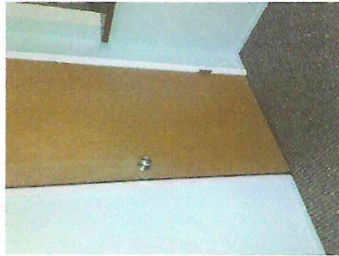
Building: Suite A 2511, Room: 33 Hall, Element Id: DRSW1-01
