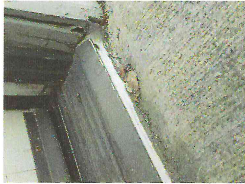
Building: Suite A 2511, Room: 25 Waiting, Element Id: DRSW1-02
